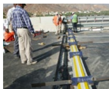
Fanja Bridge, Oman
