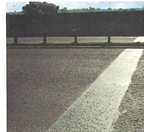
4. The finished result is a tough, long-lasting waterproof joint.
